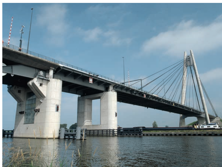
Bascule and suspension bridges
